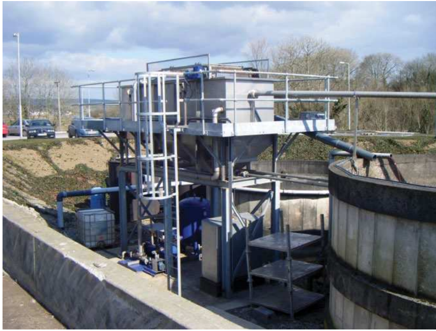
Figure 3.10 Typical DAF installation (by courtesy of Enisca, Cookstown, Northern Ireland).
