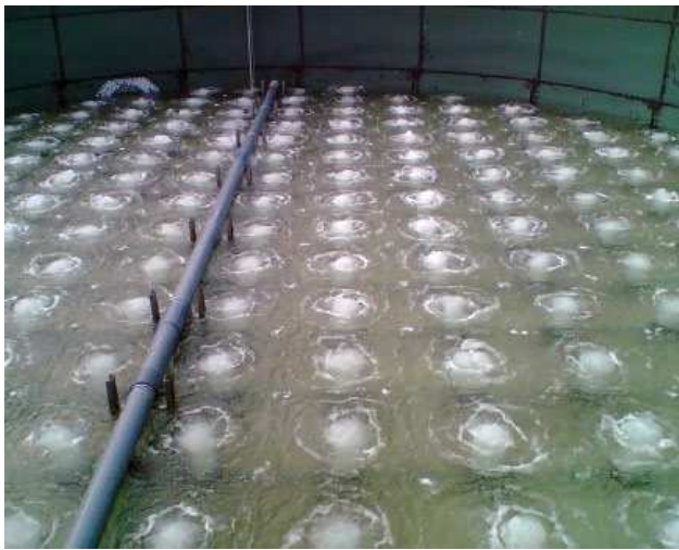
Figure 3.11 Fine bubble diffused air systems (by courtesy of Enisca, Cookstown, Northern Ireland).
