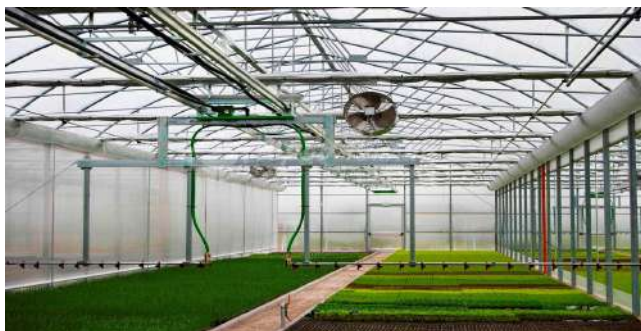
Figure 2: Modern greenhouse with improved heat circulation system
