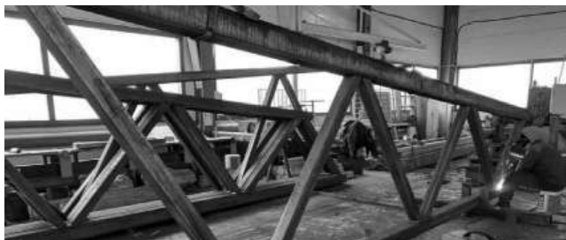
Figure-2. Surface treatment of metal structures
