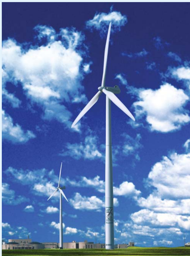
FIGURE 4.13 0.75 Megawatt generating windmills in Minnesota.
