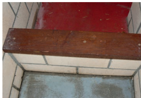
Fig. 17.8: In the large animal isolation unit, the special air lock for people is split up into two separate parts, the clean area (grey floor) and dirty area (red floor), both being separated by a bench.
