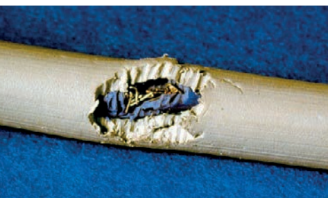
▲ Fig. 11.1: Wire that has been damaged by rats
