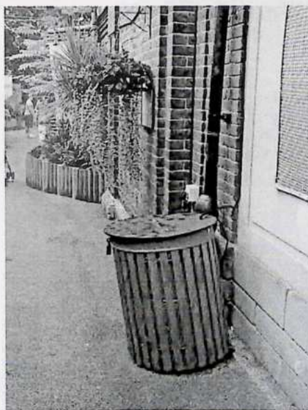
Fig. 4.5 A rainwater butt collects rain from the roof of a building at ZSL London Zoo. The rain is used to water ornamental plants.
