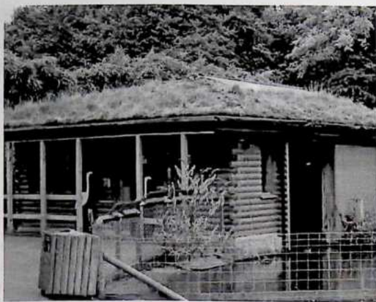
Fig. 7.40 A green roof on the flamingo house at Martin Mere (Wildfowl and Wetlands Trust).
