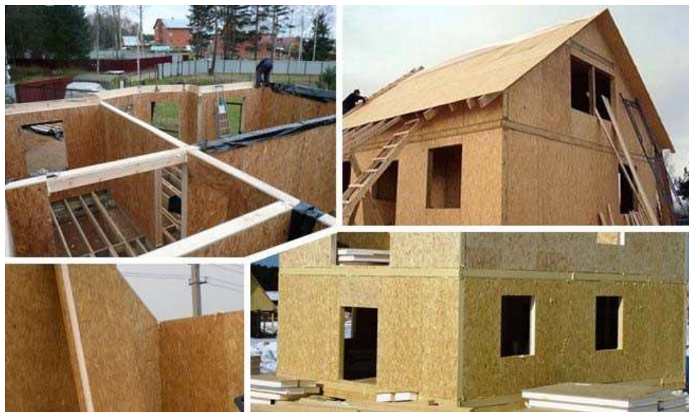
18-rasm. SIP-panellardan uy yig'ish
