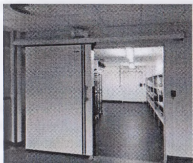
63-rasm. Polair tipidagi yig'ma sovutish kamerasing ichki ko'rinishi
