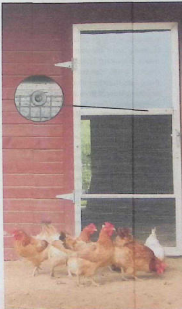
A screen door, with 1/2-inch (1.5 cm) hardware cloth secured with screws and washers, provides extra ventilation on hot summer days.
