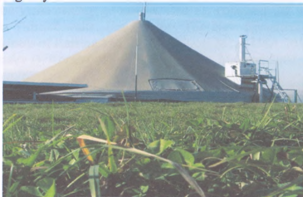
20.2-rasm. Shiqindi yoki yashil massadan biogaz olish qurilmasi.
