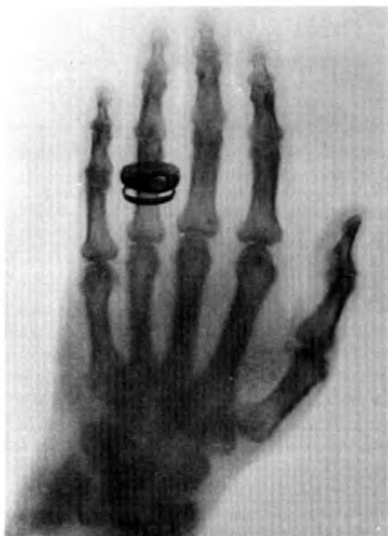
FIGURE 1.1 The first publicly taken radiograph of a living object, taken in January 1896, just a few months after the discovery of x-rays. (Courtesy of Röntgen Museum, Würzburg, Germany.)
