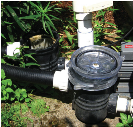
Fig. 5.3 A prefilter basket removes large particulate matter before it enters the main filter chamber, increasing the efficiency of the system.
