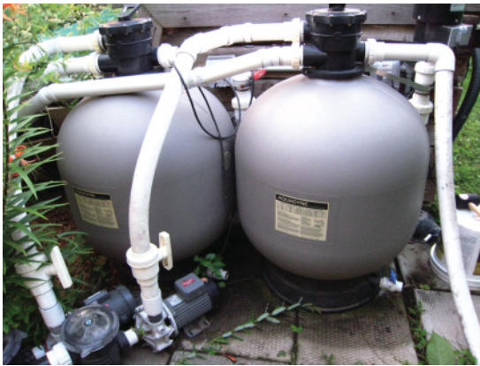
Fig. 5.2 A bubble bead filter system combines biological filtration and mechanical filtration. These two units filter 9000 gallons.
