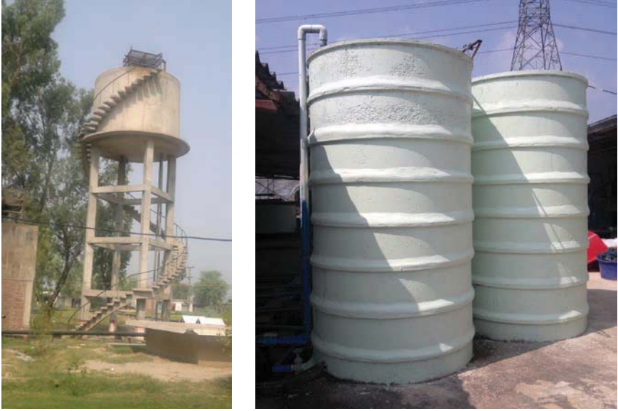
Fig. 2.7. Header tank with a filter on top that also helps oxygenate the underground water at Mian Channu Hatchery in Pakistan (left). Another header tank used for tilapia hatchery made from stacking eight large rings of concrete drainage pipes (right).
