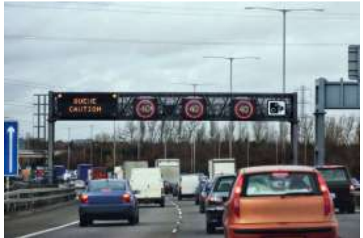
▲ Figure 5.1 Smart motorway signs
