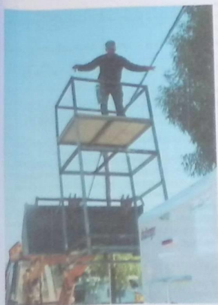
Figure 16.5 (a) Dangerous means of access with platform used to bucket of excavator. A kiss exclusively accepted in some Mexico, for good quality scaffold with protection and water, Belgium
