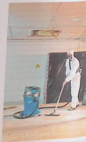
Figure 13.18 High hazard vacuum cleaner to clean asbestos material
