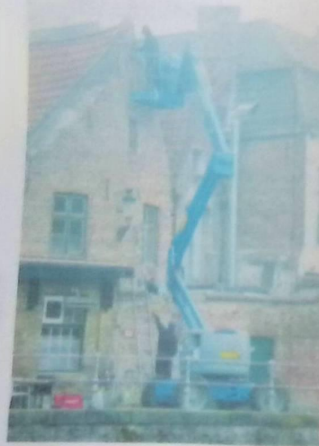
Figure 16.7 Good quality events on a lift with the covering to be used in Belgium.
