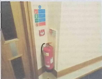
Figure 12.20 Typical fire point in offices with extinguishers, fire notices and alarm break-glass call point
