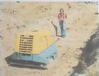
Figure 14.7 (b) Remote control vibrating plate weighing 1.2 tons with compaction in excess of a 7 ton roller which eliminates the risk of whole-body vibration. The operator is protected from vibrations, noise and dust. The machine can only be operated if line of sight is intact. In case of a loss of control the proximity recognition sensor keeps the operator safe
