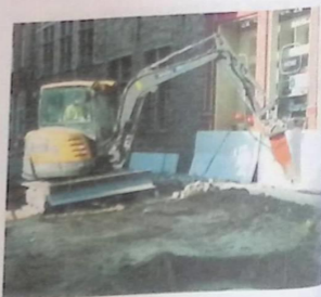
Figure 14.6 Breaker mounted on an excavator to reduce vibrations
