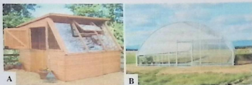
Figure 10. (A) Shed type solar greenhouse; (B) Quonset solar greenhouse [44].
